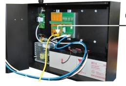
Plug the YELLOW RJ45 cable into the FIRE PANEL connection
