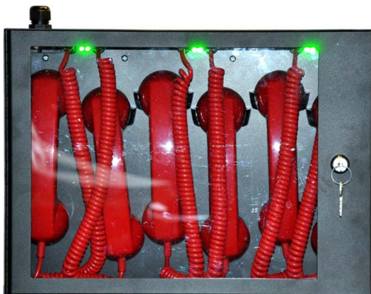
Figure 1.6 — Typical Care2 Handset Enclosure
