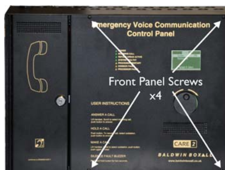
Figure 2.19 — Remove 4 x Front Panel Screws
