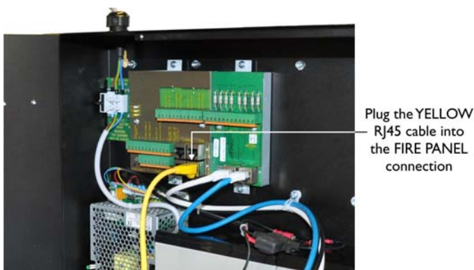
Figure 2.21 — C2CN Fire Panel Connection details
